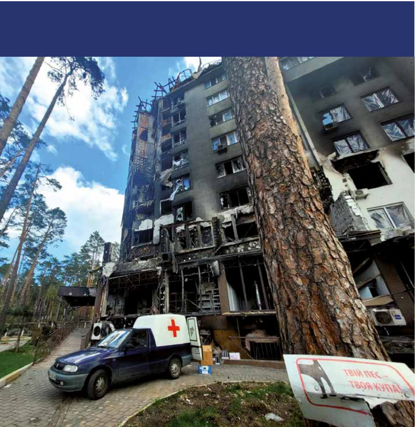
Extensive battle damage. Photo credit: Tom Garrett
